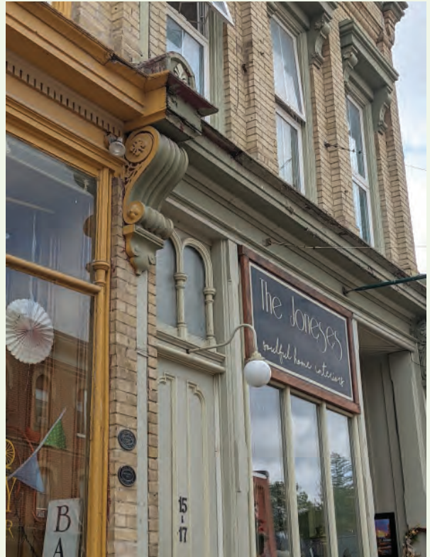
Example of fine-scale architectural details being applied to support a heritage aesthetic, such as in the downtown (guideline 103).
